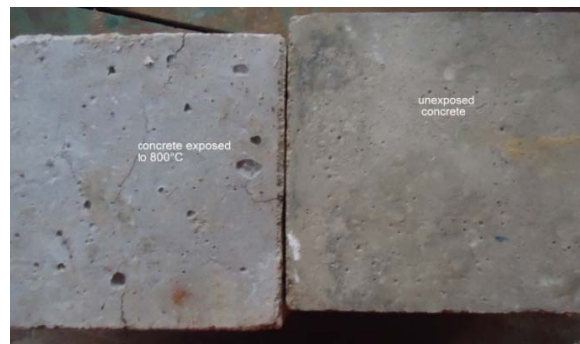
Fig. 2 Concrete exposed to 800°C
