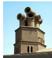
Fig. 6 Pipe Shape Wind-catchers
