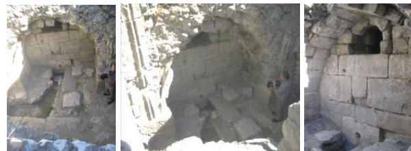
Fig. 7 Fountain's north façade
