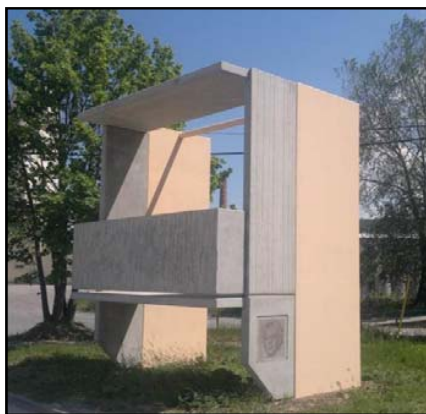
Fig. 4 Real construction of a self-supporting loggia
