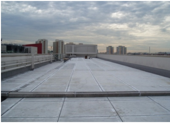
(a) Before installation of PV systems
