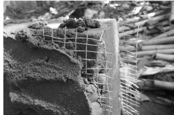
Fig. 4 Brick Wall After Applying of Ferrocement Coating
