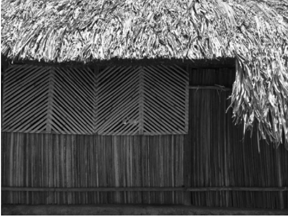
Fig. 7 Vernacular building system and materials in the sample of Pante Macassar: straw roof, palm leaves wall and window
