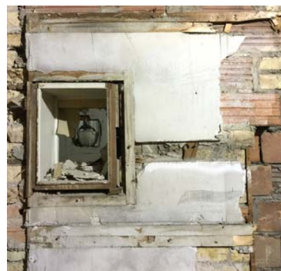
Fig. 6 An uncovered milkman delivery door, leading to center communal corridor. This has been sealed over for decades
