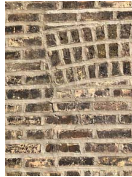
Fig. 22 Southern-facing former window opening, with toothed-in flush in-fill brick; this modification was done sometime prior to the conversion of the apartment building into a museum
