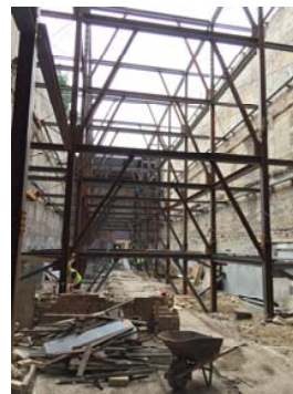
Fig. 19 Newly installed structural steel frame. Portion of old brick wall is still visible in the foreground
