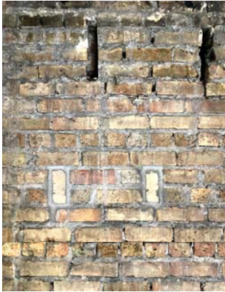
Fig. 20 The very rough inside face of an existing perimeter three-wythe thick masonry wall, with as-yet-to-be filled joists pockets
