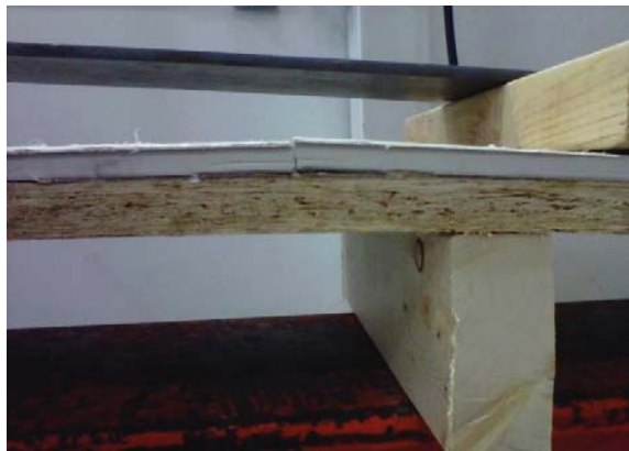
Fig. 11 Tensile crack in the overlay on top of the intermediate supports (negative bending moment)
