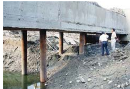
Fig. 1 Example of embankment failure by piping
