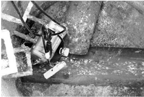
Fig. 1 Equipment setup in a sewer manhole chamber
