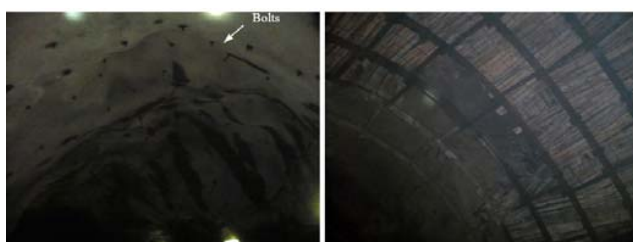
Fig. 2 Places with reinforced support in the ramp
