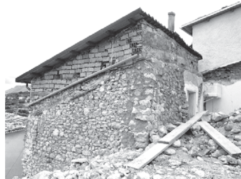
Fig. 3 Typical residential building
