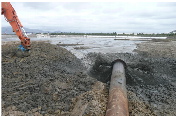
Fig. 4 Dredged material placement into port's ERA - 2011
