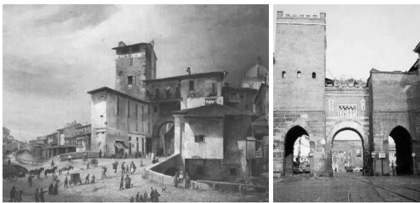
Fig. 1 Milan, current and historical view of Porta Ticinese, strongly influenced by the “liberation restoring” of Camillo Boito
