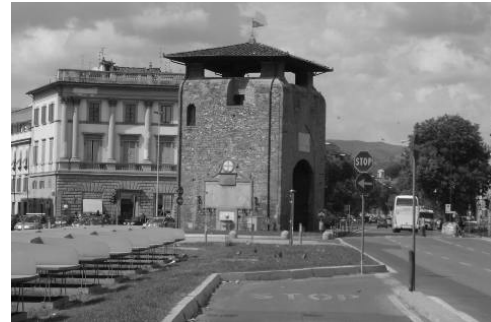
Fig. 2 Florence, Ancient city door in Piazza della Libertà, after the demolition of urban walls
