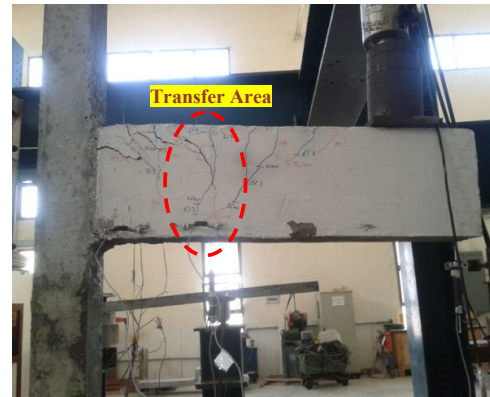
Fig. 15 Cracks at the failure of SP4
