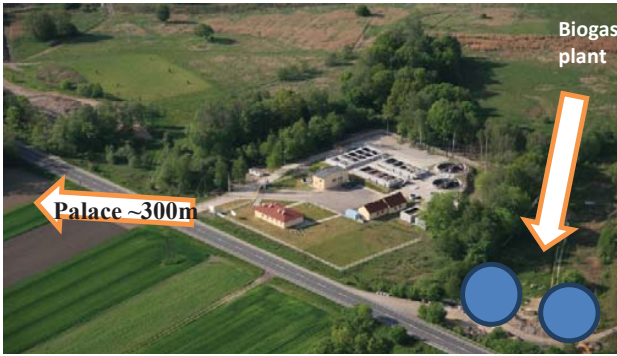
Fig. 7 Wastewater treatment plant with a biogas plant
