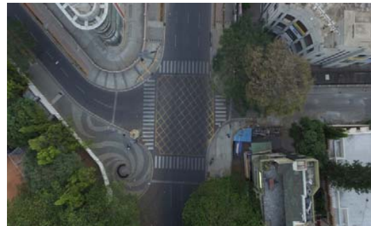
Fig. 4 Tender SURE infrastructure at Richmond road, Bengaluru
