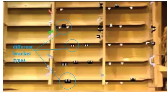
Fig. 4 Located brackets on the screen
