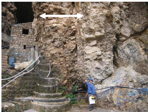
Fig. 5 Fractured zone of CBF
