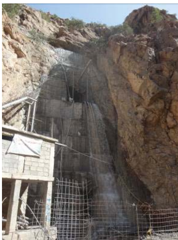
(b) After plugging
