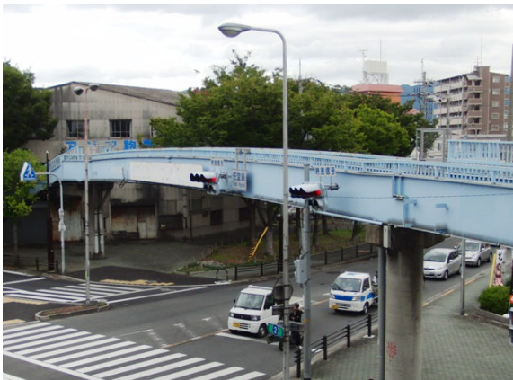
Fig. 13 Pedestrian bridge being tested
