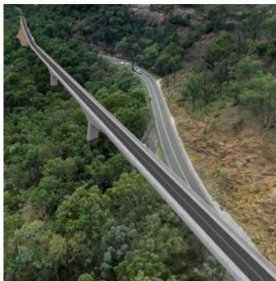
Fig. 7 Completed bridge in relation to existing road
