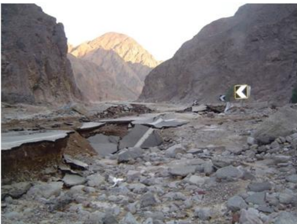
Fig. 2 Sever flash flood impact on the international road
