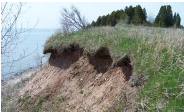
Fig. 2 Collapse of layer undercut by piping / sapping [6]
