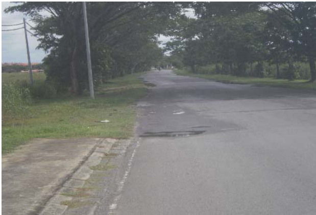
Fig. 1 The road section at Curtin entrance
