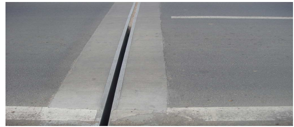
Fig. 4 (b) Losing of joint material
