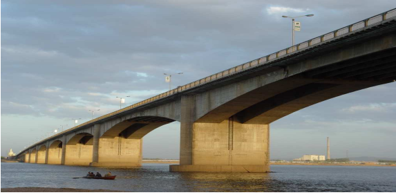
Fig. 1 (a) View of spans
