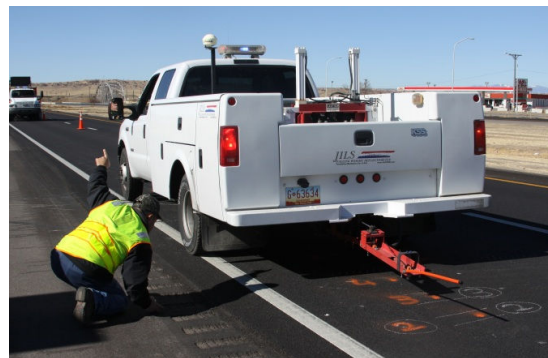
Fig. 1 Execution of FWD test
