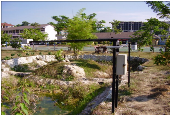
Fig. 3 Rainfall and Water Level Station
