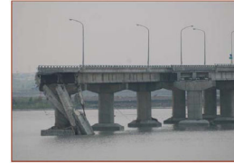
Fig. 18 Case 2: the bridge failure in flood
