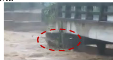
Fig. 19 Case 3: the bridge failure in flood
