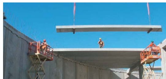
Fig. 1 Assembling roof panels.
