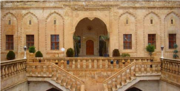
Fig. 8 Facade of Mardin PTT House
