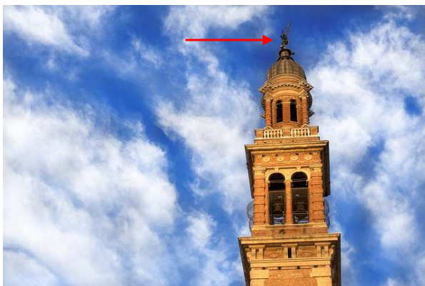
Fig. 2 The bell tower of Lendinara; the red arrow evidences the location of the anemometer
