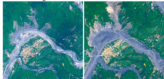
Fig.1 Baolai-2 Bridge and its surroundings before and after Typhoon Morakot strike
