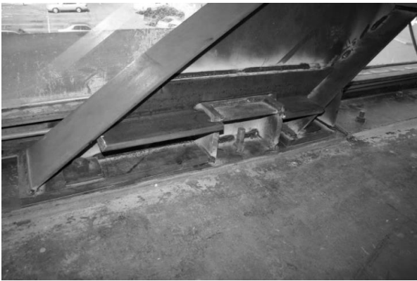
Fig. 13 Photo of constructed shearlink
