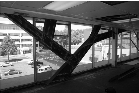
Fig. 14 Photo of frame under construction
