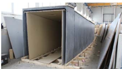
Fig. 13 Removing of wooden formwork
