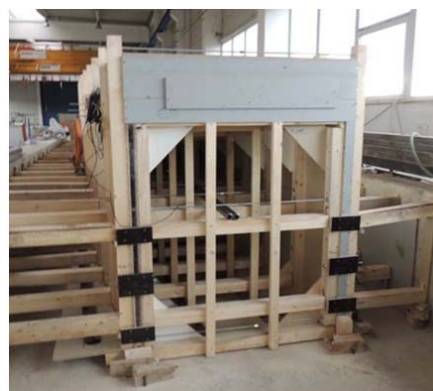
Fig. 16 Formwork of footbridge II
