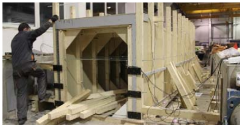
Fig. 12 Wooden formwork of footbridge I
