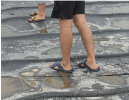
Fig. 10 Ground in half way of foundation treatment
