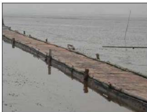
Fig. 3 Complete floating bridge
