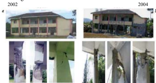
Fig. 10.a.Severe Cracking and Damage to soft first storey columns of Nabagram Panchayat Bhavan building primarily due to 'missing' ties in 2002 earthquake, b.more damage in 2004 earthquake to same columns which were 'retrofitted'[9].
