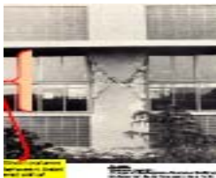
Fig.4. large window openings AND SHORT COLUMN
