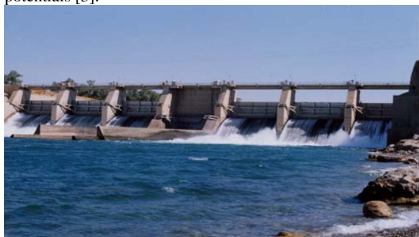
Fig. 1 The Dez regulating Dam with 13000 million cubic meters reservoir
