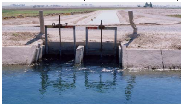
Fig. 3 A cross-regulator in a main canal
