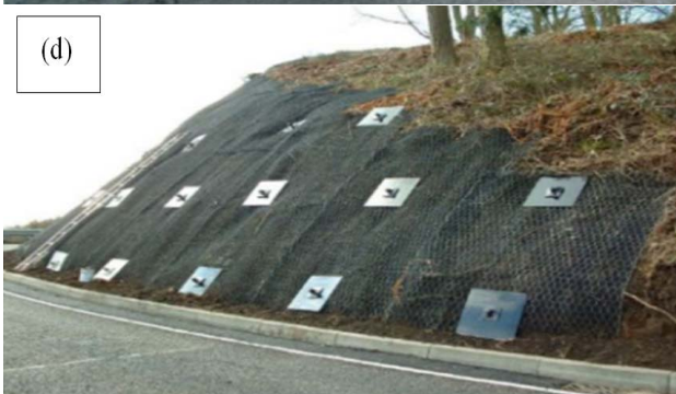
Fig. 5 Soil Nailing Method
