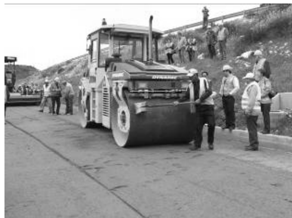
Fig. 3 Roller compacting SFR-RCC layer during demonstration day.
