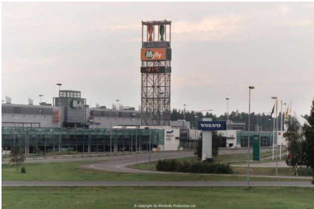
Fig. 5 Couple of WS-12 VAWT at the shopping center “Mylly”, Raisio, Finland (from: [19]).
