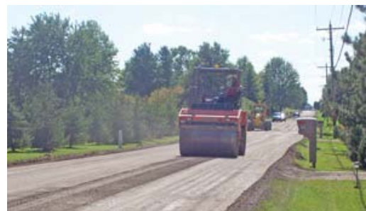
Fig. 3 Compaction of FDR base layer
