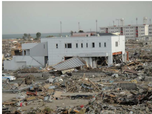
Fig. 11 Steel structure almost intact
