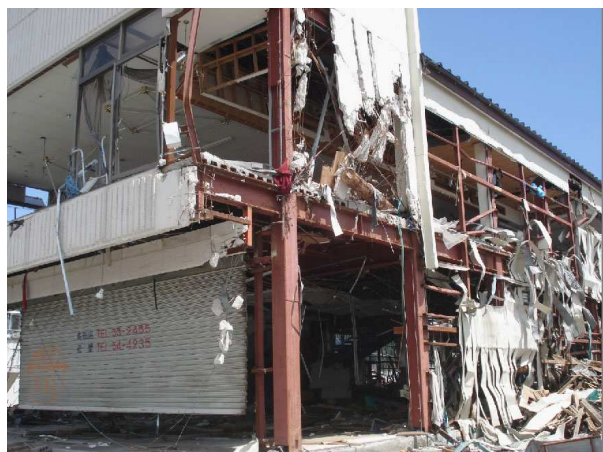
Fig. 12 Destruction of panels
