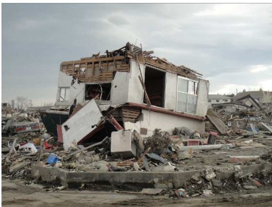
Fig. 10 Over turning of upper floors
