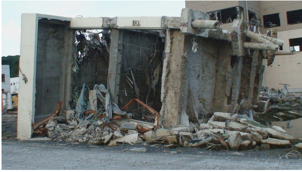
Fig. 23 Collapse of 2 story RC building
