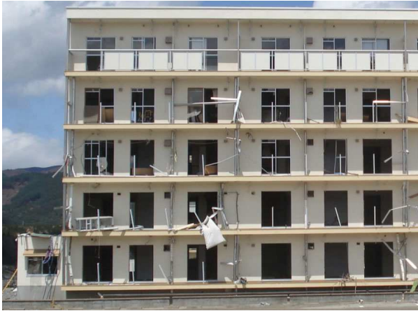
Fig. 18 Detail of damages on balconies
