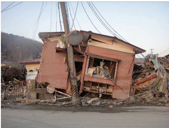
Fig. 9 Transportation of the upper floors
