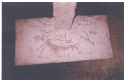
Fig. 2 Crack pattern as exhibited by Se-12
