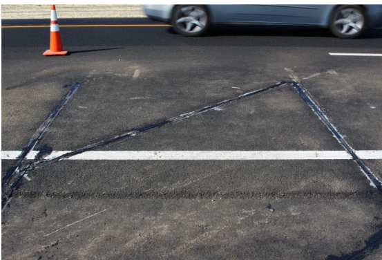
Fig. 5 Installation of axle sensing strips
