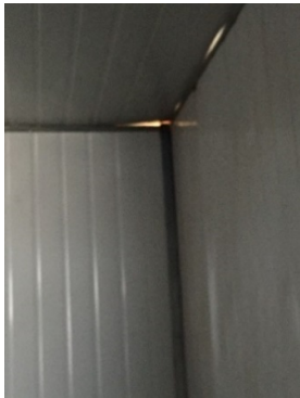
Fig. 5 Gaps between junctions [13]
