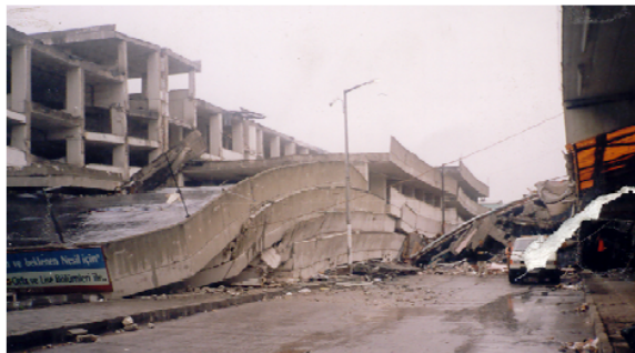
Fig. 1 A seriously damaged RC building in Marmara region
