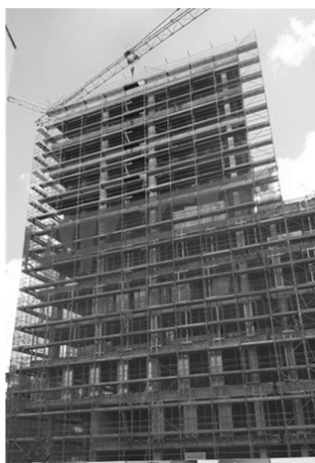
Fig. 1 A view of the scaffolding
