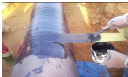
Fig. 6 Wrapping process of Kevlar tape repair system
