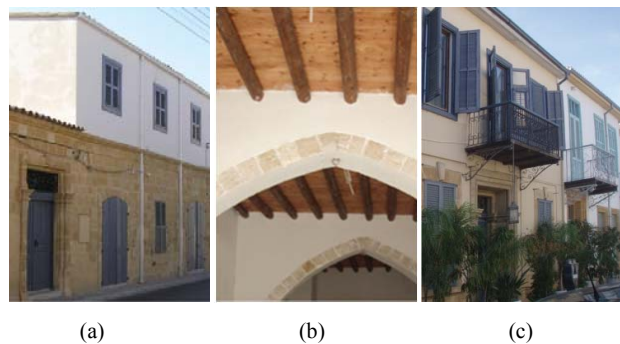
Fig. 10 (a) Load bearing stone and mud-brick walls, (b) Traditional flat roof, (c) External shutters in windows of traditional buildings
